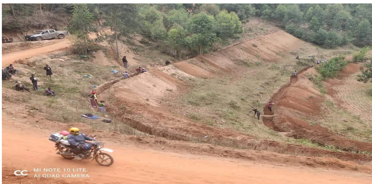
Figure 14: Road Improvement Programme in Mbooni Sub County
