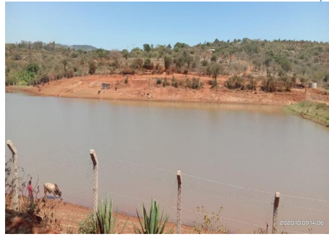
Figure 13: Katilini Earth Dam
