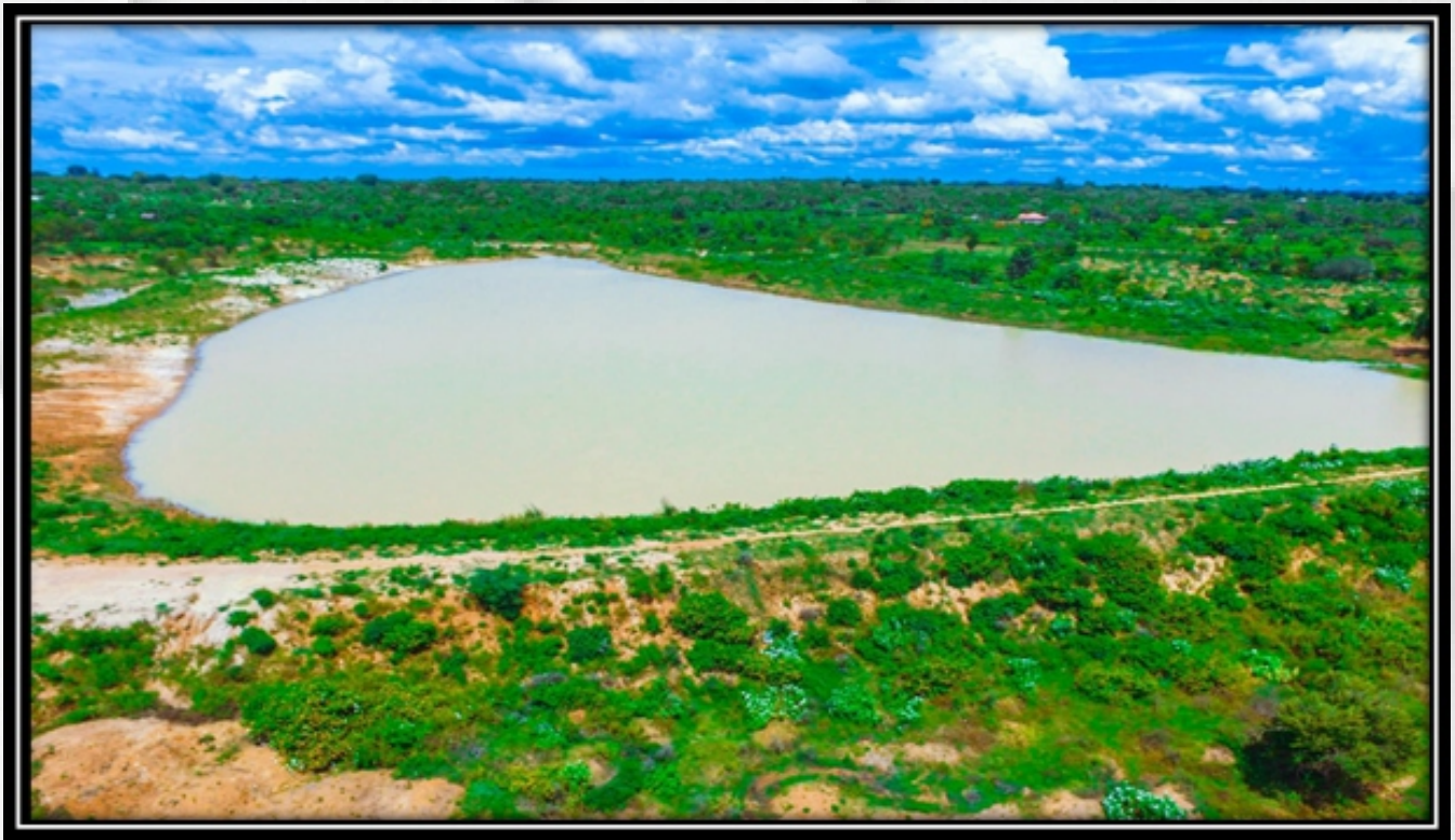
Figure 7: Kyamakuthi earth dam in Kalawa with capacity of 47,233M3. The project serves approximately 10,000 people and 25,000 livestock with reliable water throughout the year
