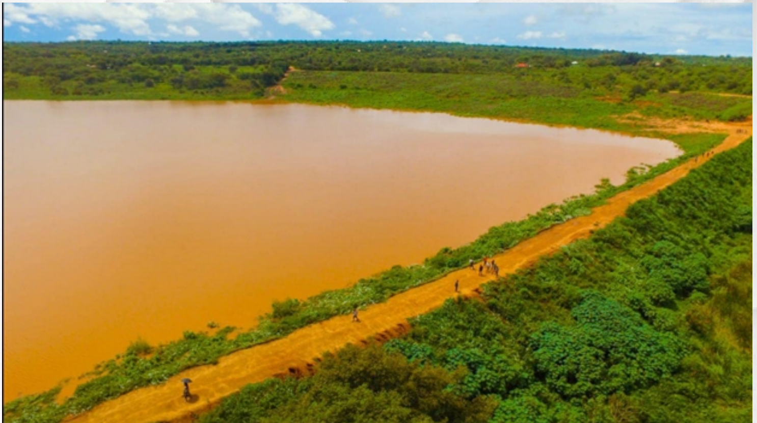
Figure 8: Ndukuma Earth Dam In Kikumini/Muvau Ward Is A Flagship Project Earmarked For Distribution In FY 2024/25
