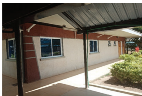
Makueni L5, CTScan. Light colored walls with shading & e-coated windows
