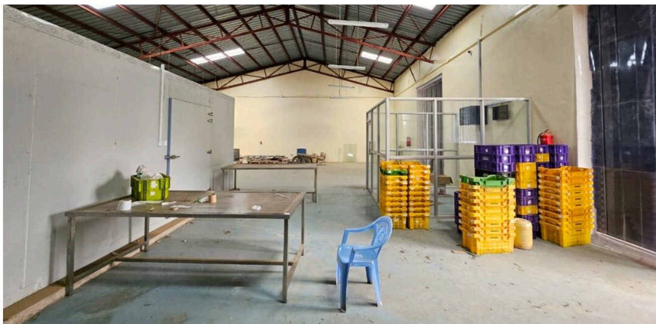
Kilungu cold room not operational due to lack of power, water and PMC operationalization. (Photo: WRI)
