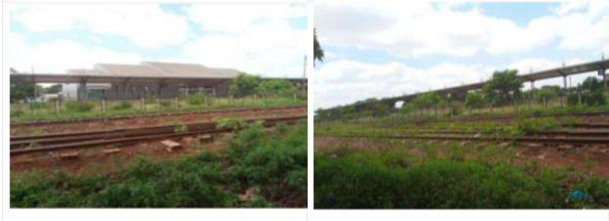
Figure 16: Emali SGR terminus and SGR & Old Railway line in Emali
