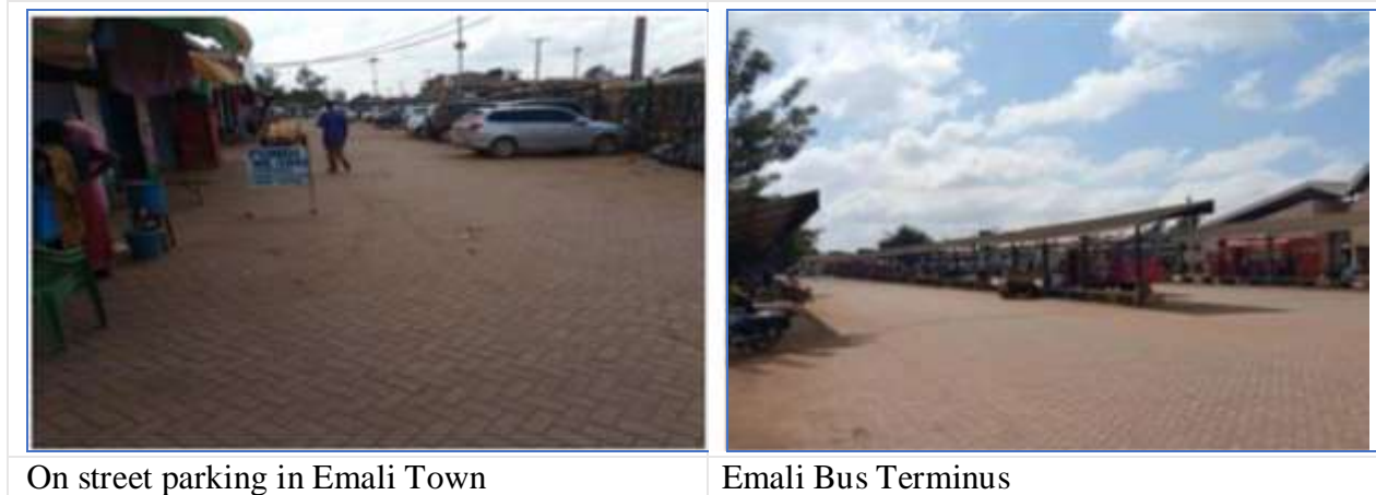
Figure 12 b: Several Road Infrastructure in Emali and Sultan Hamud Towns
