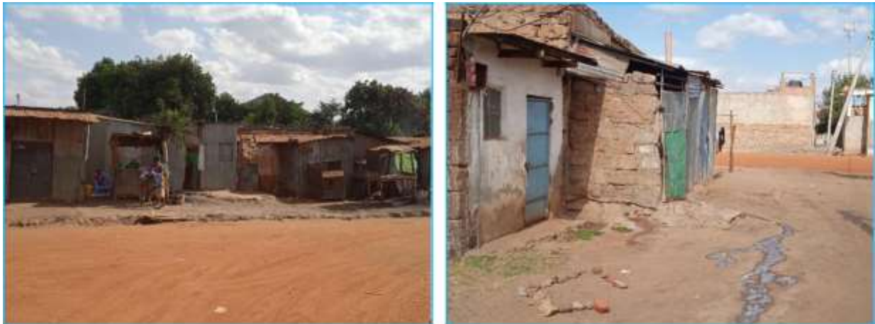
Dilapidated houses in Sultan-Hamud town
