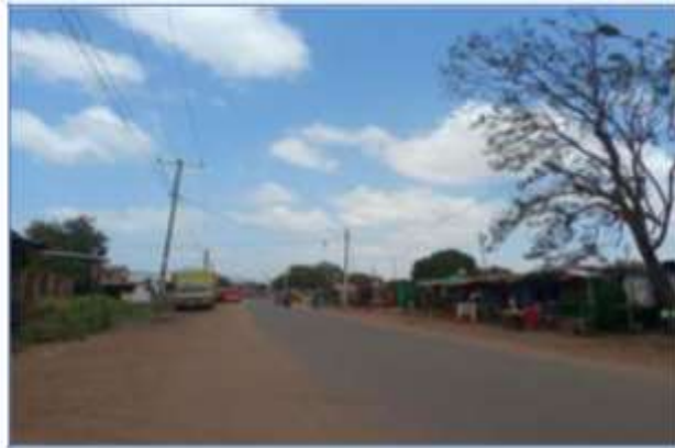
A street in Emali Town paved and providing for wayleave
