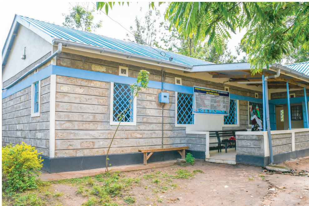
Renovated - Kee Model Facility
