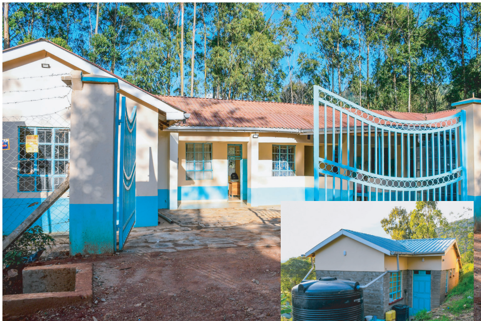
Utangwa Dispensary renovations and stuff house
