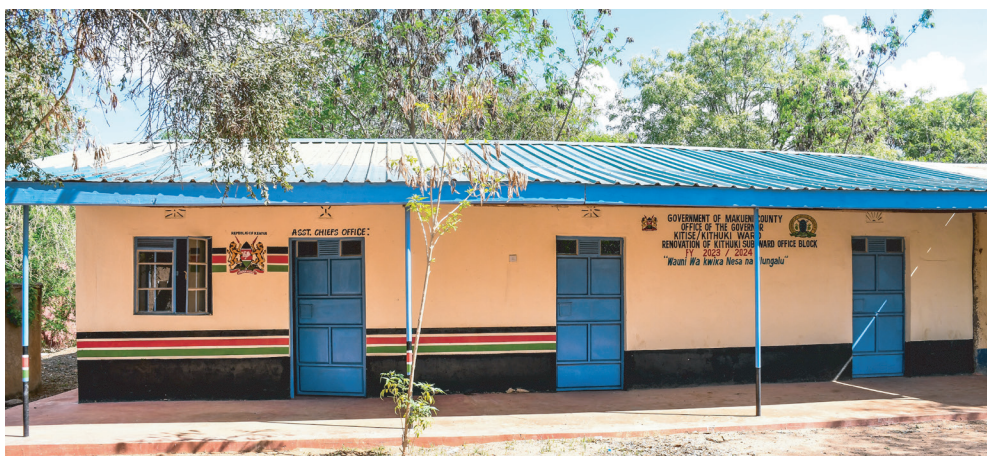
Renovated Kithuki Village Administrator's Office
