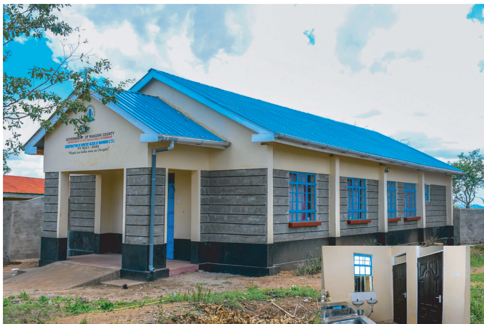
Mavindini CTTI Dormitory
