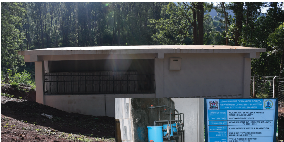
Mulima Treatment Plant
