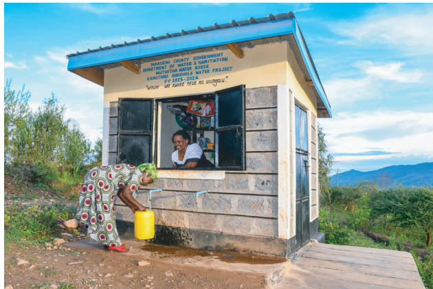
Kamuthini Borehole (Muthitha Kiosk)
