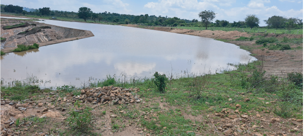
Ngosini Concrete Dam
