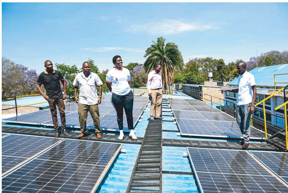
Solarization at Makueni County Referral Hospital
