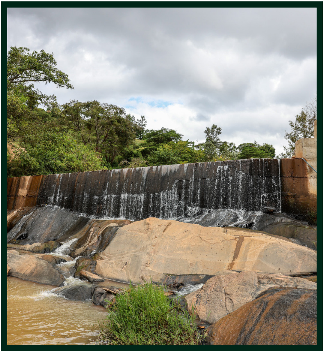
Wautu-Kyangati sand dam, built along Wautu river to provide water for domestic use and irrigation. It is also an environmental restoration project.
