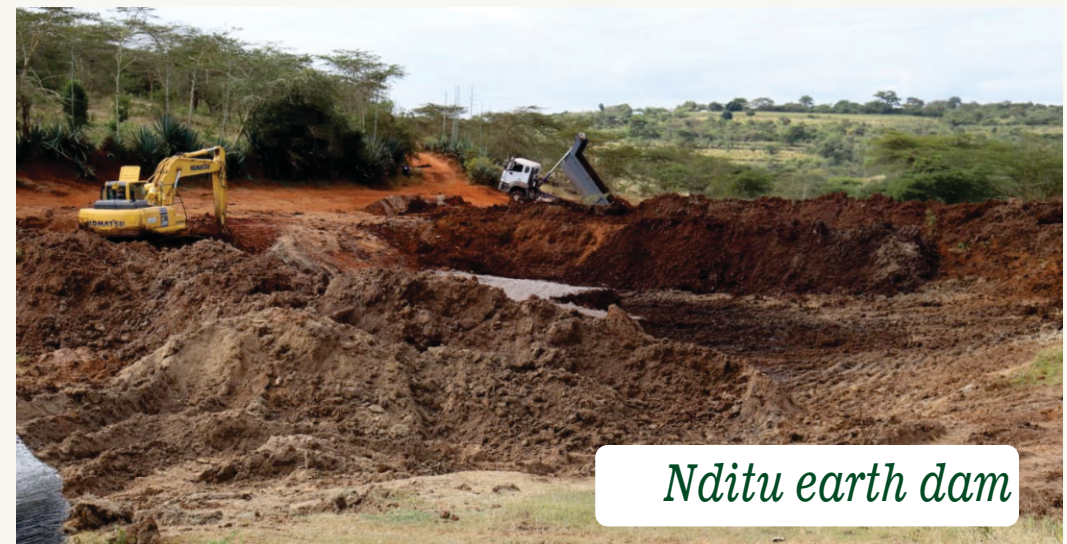
De-silting Nditu earth dam
