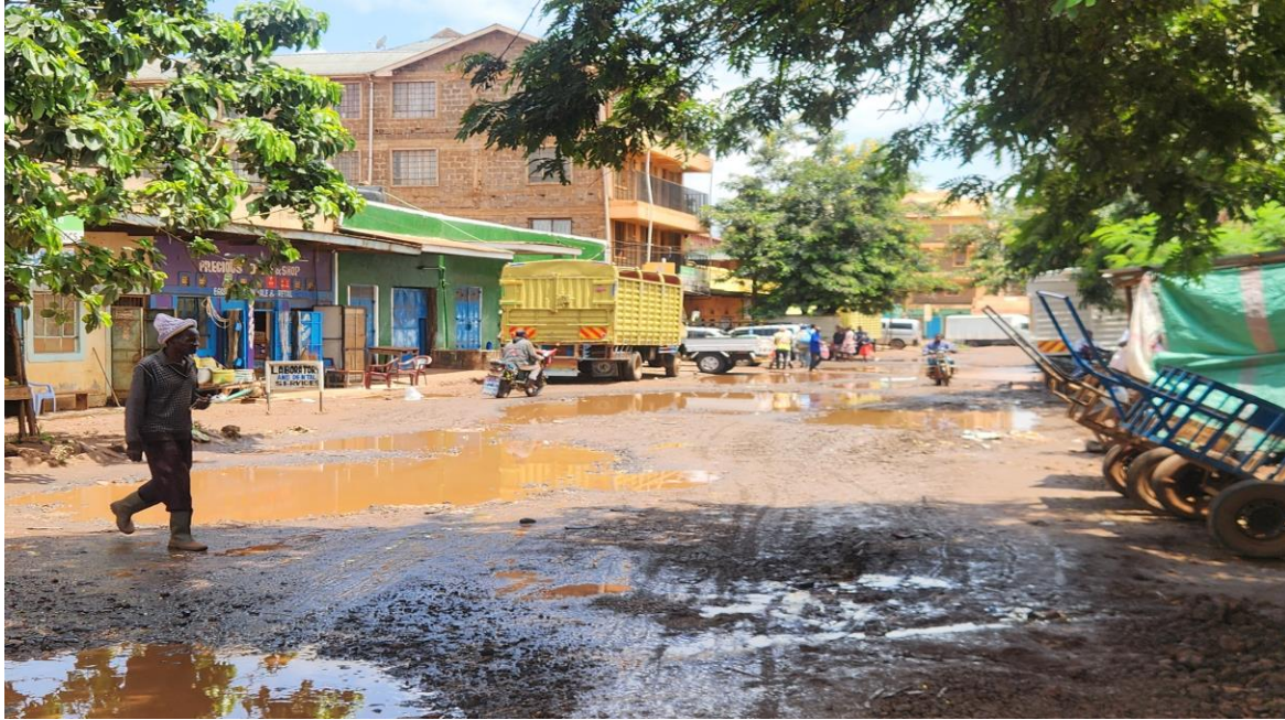
Poor storm water drainage – Emali Town
