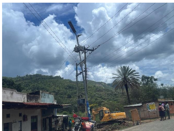
Solar Street light at Muangini shopping Centre
