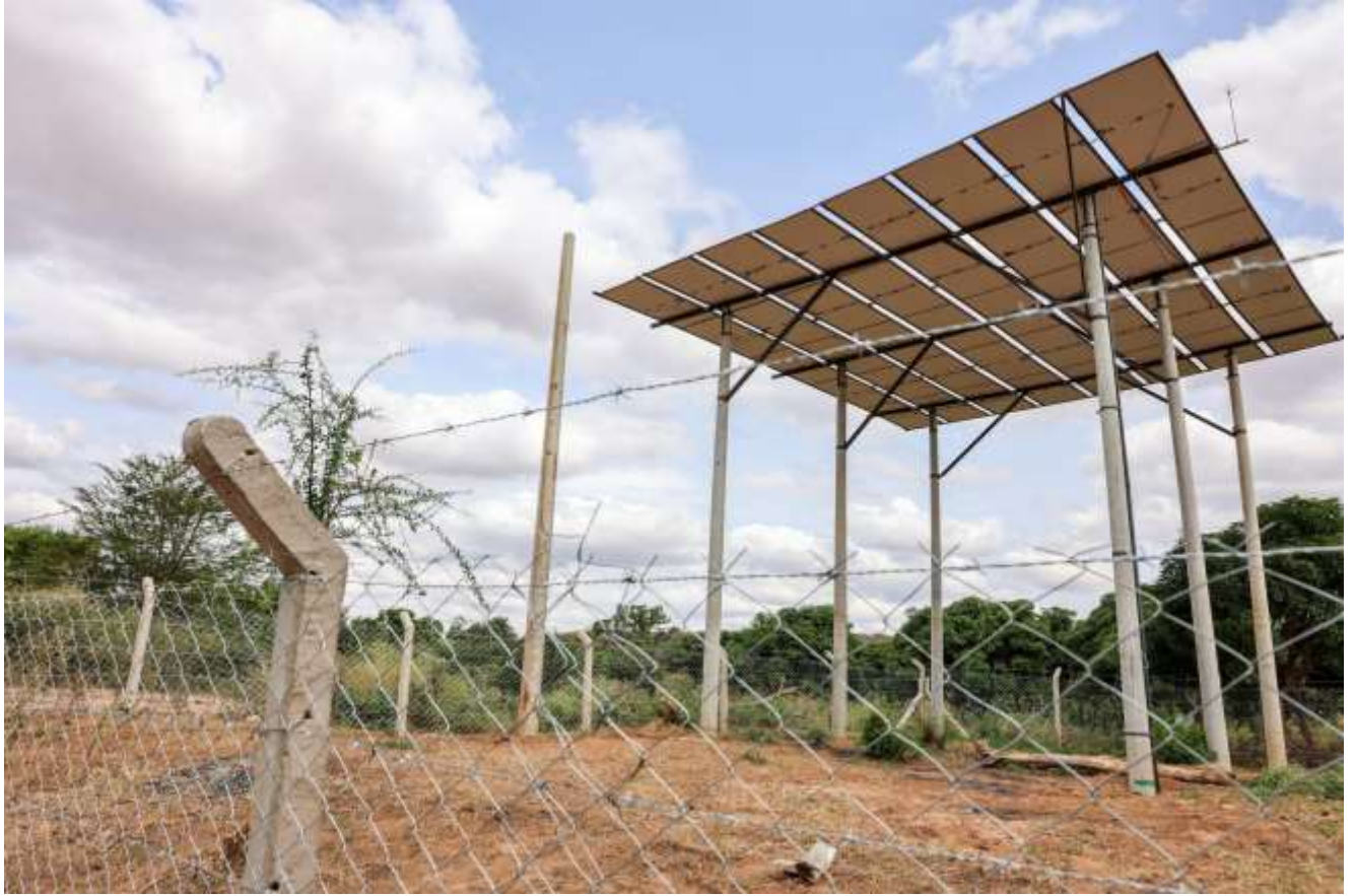
Figure 11: Elevated positioning of solar panels in projects
