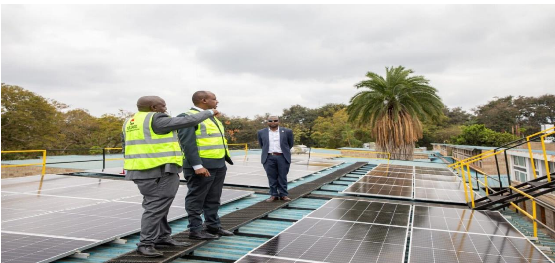
Figure 16: 205kWp grid-tier Solar System in Makueni Referral Hospital
