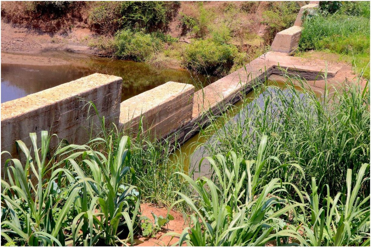
Figure 8: Sand Dam at Kalamba
